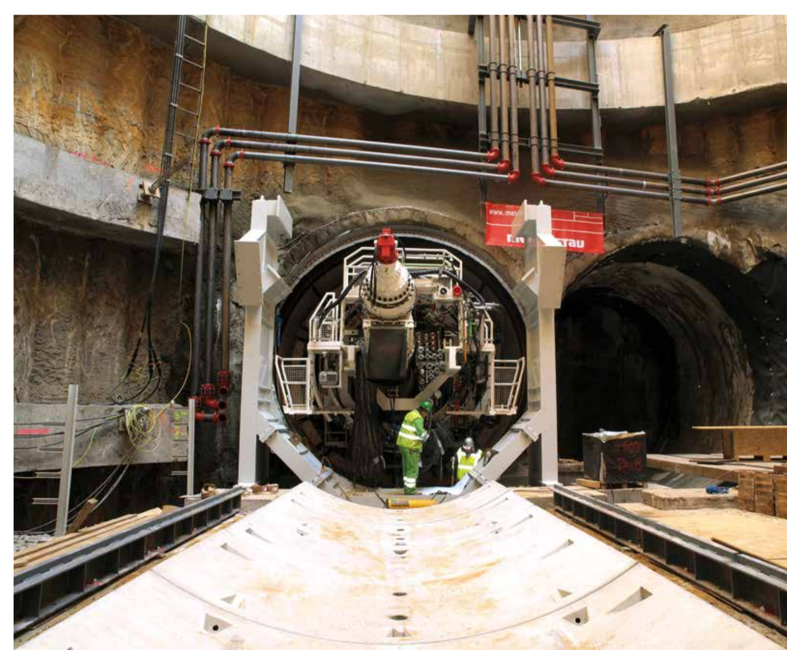
Instalace razicího štítu v pažené jámě – prodloužení metra A – archiv Metrostav Praha Installation of the TBM (tunnelling boring machine) in a sheeted foundation pit – extension of the Metro line A – Metrostav Co. archives, Prague, the Czech Republic
