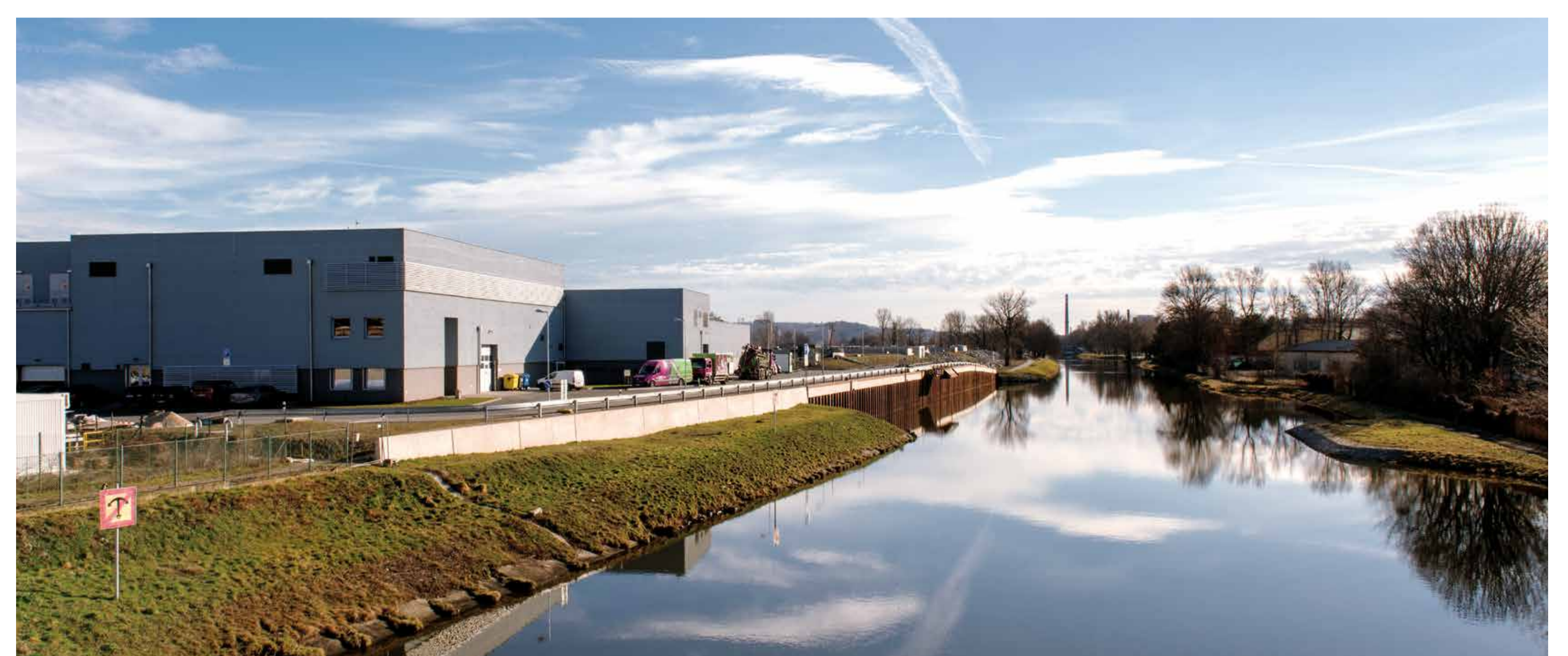
Pohled na Novou vodní linku ÚČOV Praha View to the New Water Line of the Central Wastewater Treatment Plant in Prague
